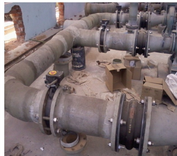
FRP Pipe Erections
